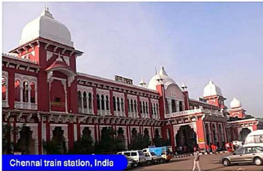
Chennai train station, India
