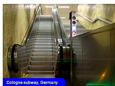
Cologne subway, Germany
