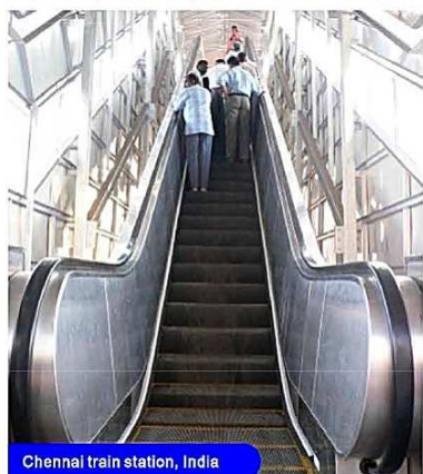
Chennai train station, India
